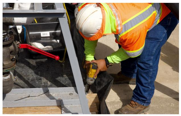
Civilian personnel assigned to Joint Task Force-Red Hill (JTF-RH) secure a fuel pump in preparation for draining the surge tanks at the Red Hill Bulk Fuel Storage Facility (RHBFSF) on Joint Base Pearl Harbor-Hickam, Honolulu, Hawaii, July 25, 2023. US Marine Corps Photos
